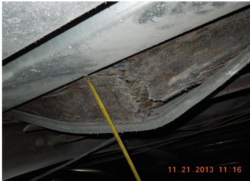
Figure 5.22 - Large lagging deflection (8") due to a pointed impact
