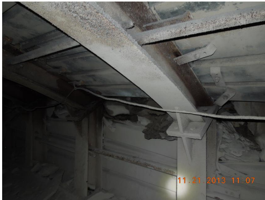
Figure 5.19 - Steel sets under the secondary roof fall area
