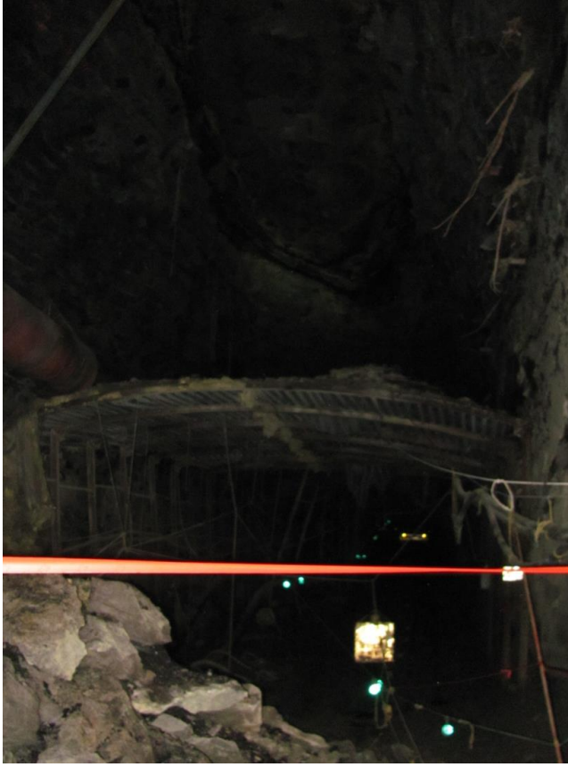
Figure 6.2. Large roof fall cavity
