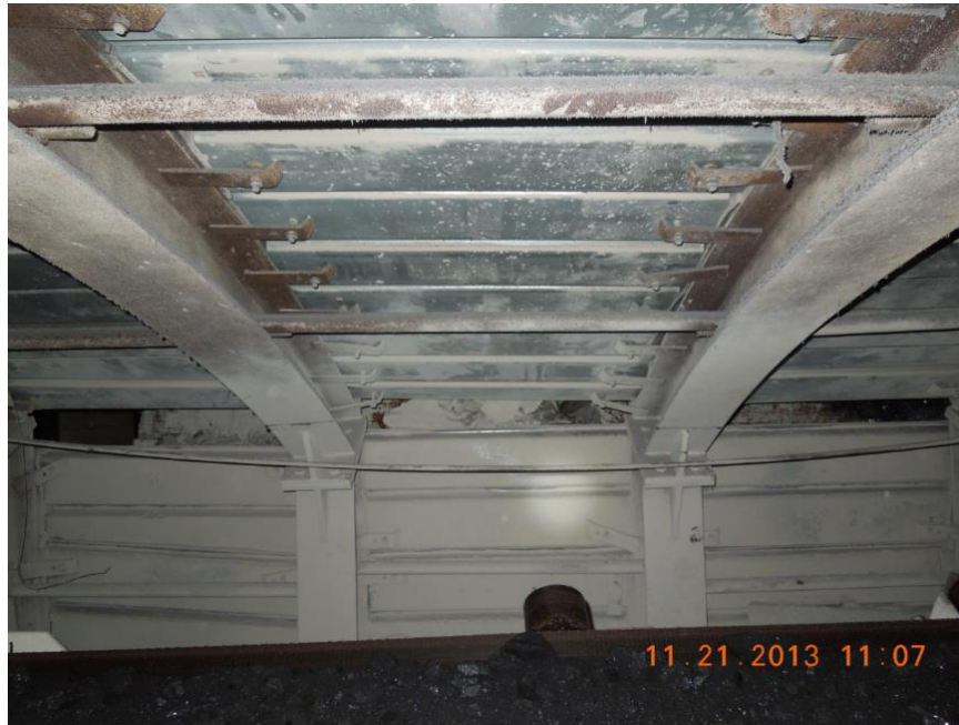
Figure 5.18 - Steel sets under the secondary roof fall area
