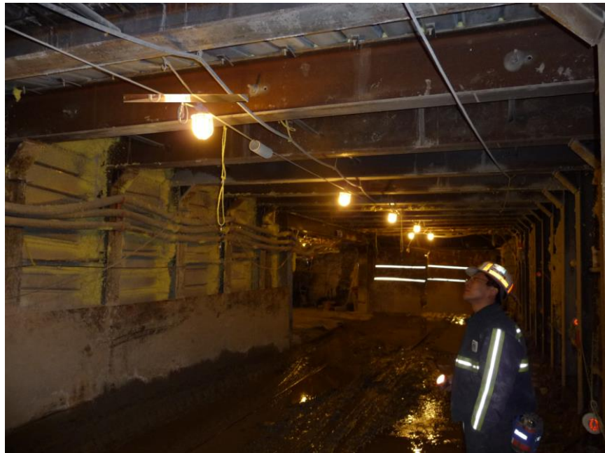
Figure 6.11. Rehabilitated slope bottom
