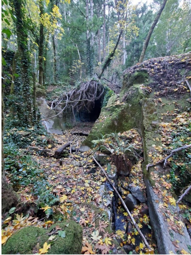
Figure 12. Wrights tunnel entrance as it stands today (S. Brewer)
