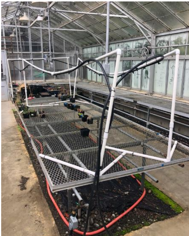
Appendix H. The automatic watering system in the HSU Experimental Greenhouse. Photo taken on September 25, 2020 by Sam Kelly.
