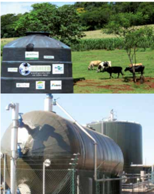
Figure 5 Upflow (top picture) and plug (lower picture) flow examples of digesters (Photo: Top: ITAIPU Binacional, Brazil; Bottom: Marches Biogas)
