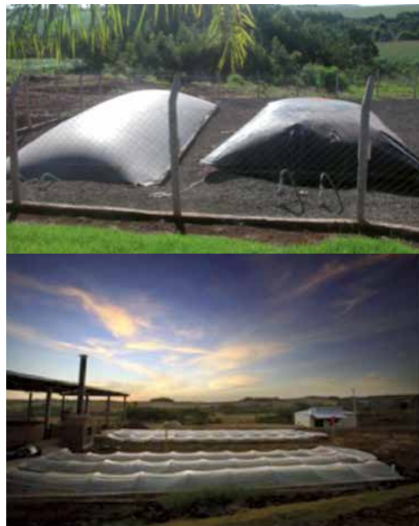
Figure 6 Lagoon and bag type digestion systems (Photo: top: C. Lukehurst; bottom: C. Bley)
