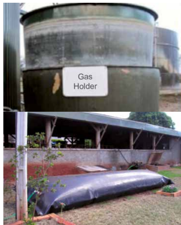
Figure 9 GRP bell-over-water gas holder (top) and simple gas bag storage at a Brazilian farm (bottom) (Photos: A. Bywater (top); D. Baxter (bottom))
