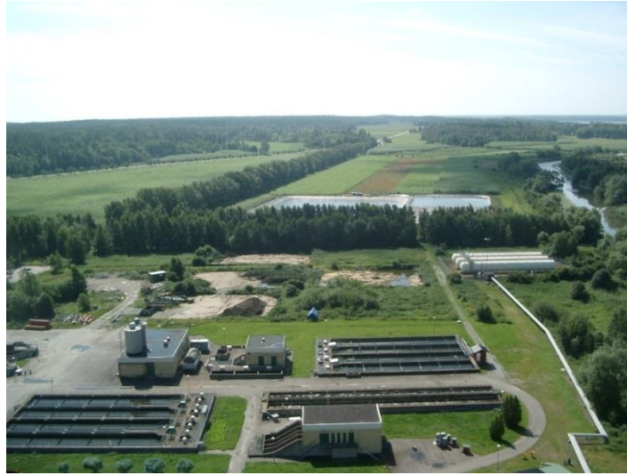
Figure 5.14. View of a municipal wastewater plant in Enköping, Sweden, with water storage ponds and (behind the ponds) the willow fields that are used as vegetation filters. The photo is taken from the roof of the heat and power plant that uses the locally produced biomass (Photo: Pär Aronsson, SLU).
