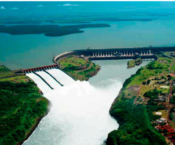
Figure 4. Water being bypassed at the hydro-electric power plant in Itaipu with a capacity of 14GWe
