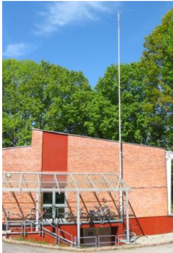
Fig. 2: the laboratory for greenhouse gas concentration monitoring (Bd 5). Air is sampled from the 15m high mast.
