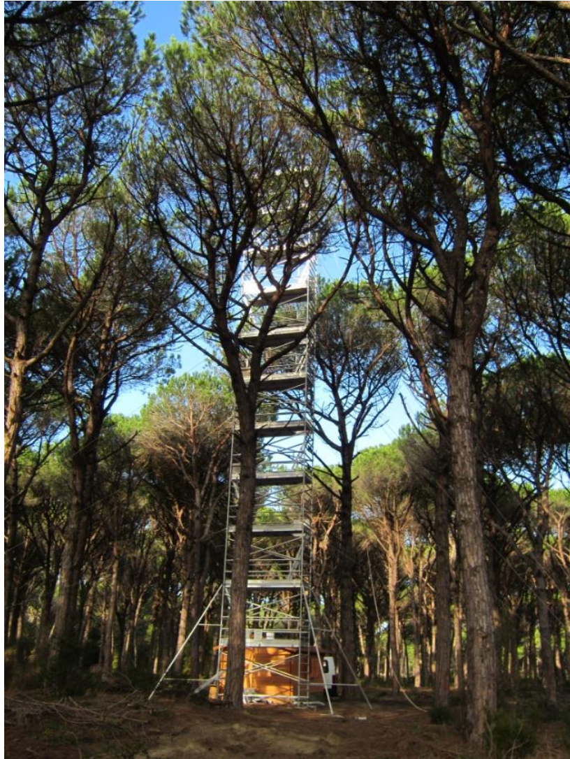
Fig. 61: Newly erected tower at the pinus pinea site that will hold the measurement equipment.
