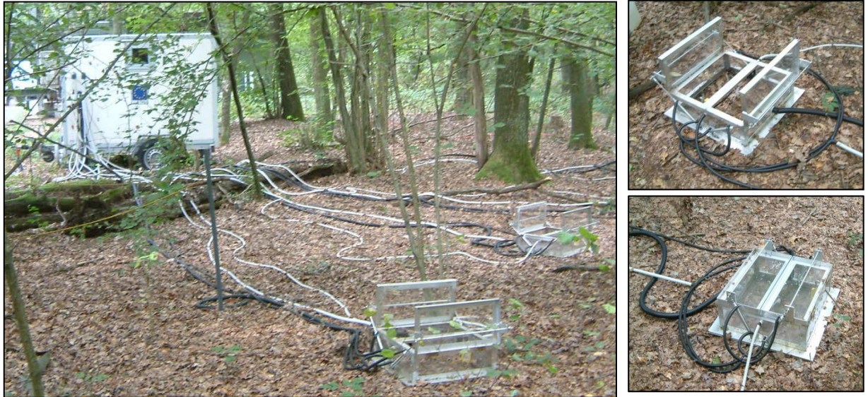
Fig. 53: Chamber system to measure NO & NO 2 fluxes from soil at the ABC-IS forest flux site.
