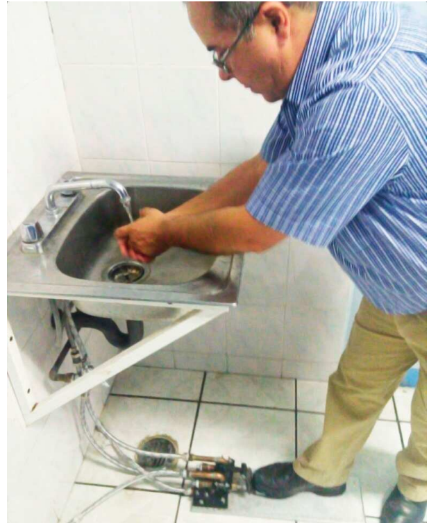
Figure 6. Pedal-operated wash basin (BRUNOTICIAS, 2017).
