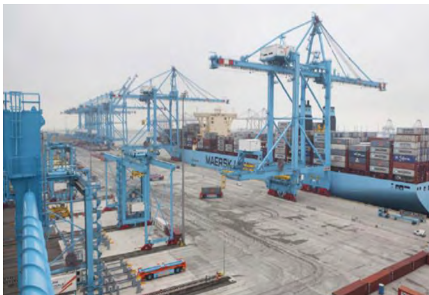
Figure 4. Maasvlakte II Terminal at Port of Rotterdam
