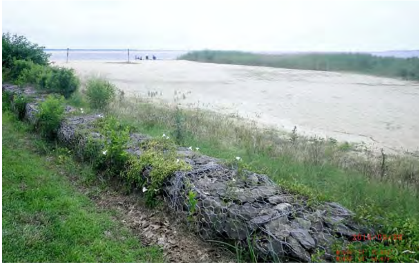
Gabion basket wall along the road behind BW 1.
