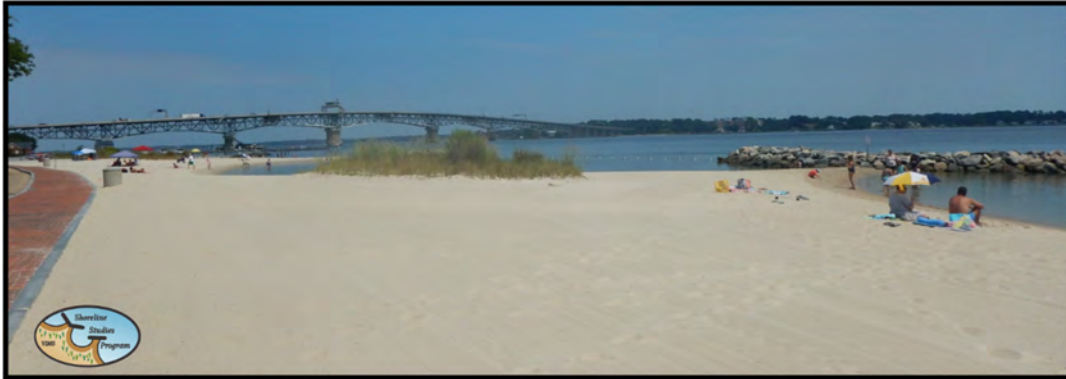
Figure 4-2-4. A wide recreational beach exists at Yorktown Beach shoreline on 31 Jul 2019. Though the backshore is low, the beach provides protection to upland structures.
