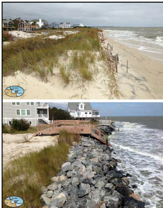
Figure 4-5-4. Top: Northern section of the Bavon reach during a high water event on 5 October 2015. The wide dunes protect the houses. Bottom: a revetment was constructed because the dunes had eroded along the southern section of the reach but no beach
