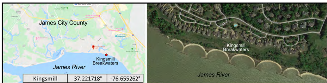
Figure 4-4-1. Left: Location of Kingsmill breakwaters, and Right: Google Earth image of breakwaters taken in May 2018.
