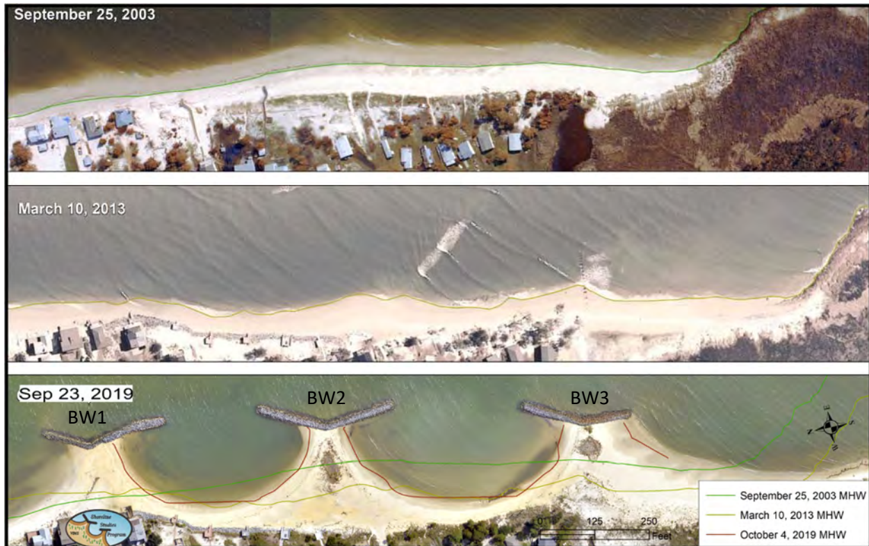
Figure 4-5-6. Shoreline change between 2003 and 2019 at the Yorktown breakwaters. The 2003 and 2013 shorelines are approximately mean high water based on the digitizer's best guess of the features shown on the aerial photo. The 2019 shoreline is from the survey data.
