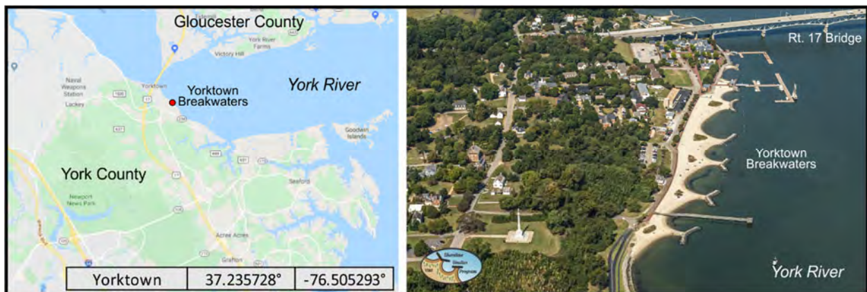
Figure 4-2-1. Left: Location of Yorktown Beach breakwaters, and Right: Aerial image of breakwaters taken on 23 Sep 2019.
