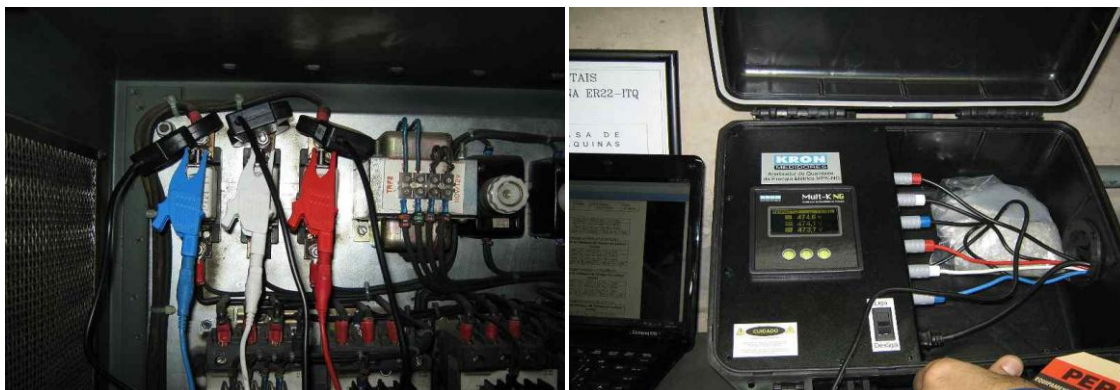
Figure 3 - Installation of Power Analyzers Panel of ER 22 and ER 28
