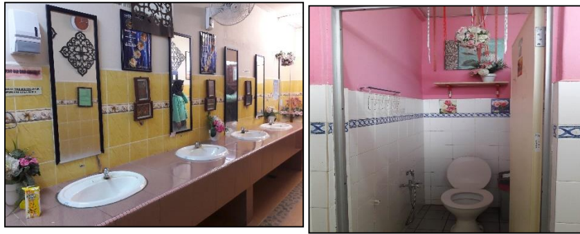
Fig 4. The condition of toilet in DC
