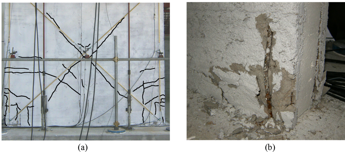
Figure 4. (a) Horizontal, vertical and shear cracking at peak lateral load. (b) Disintegration of concrete and bar buckling at the base of panels.
