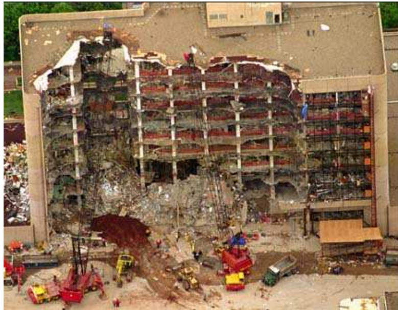
Figure 5.2. Alfred P. Murrah Federal Building [60]
