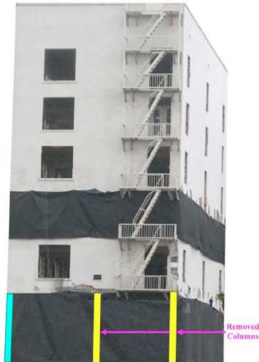
Figure 4.12. South-east view of the Hotel San Diego (from Sasani and Sagioglu [62])
