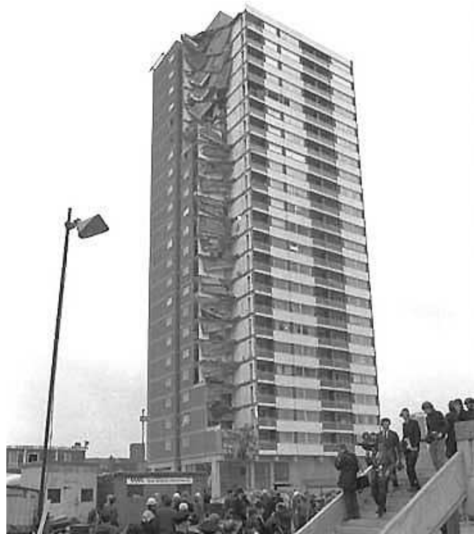
Figure 5.1. Ronan Point Apartment after collapse [16]
