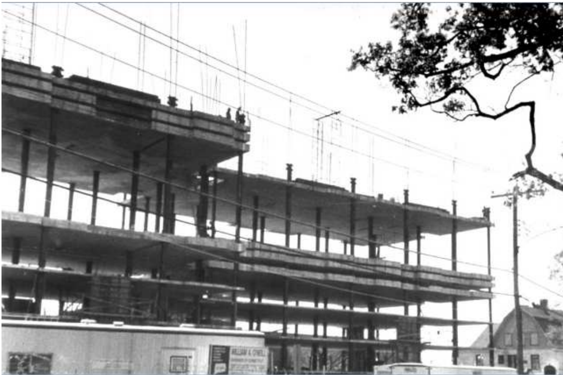
Figure 5.4. L'Ambiance Plaza during the construction phase [22]
