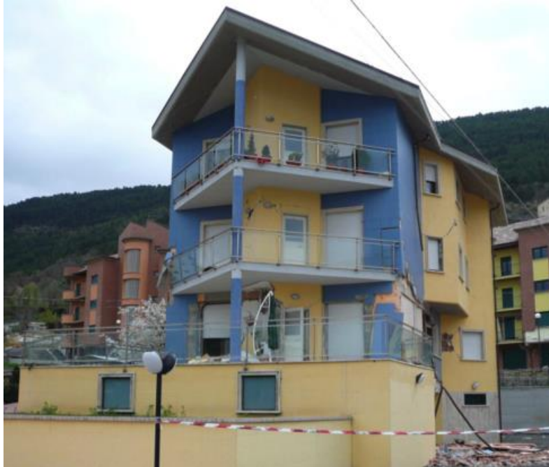
Figure 24 - Damage for torsional effects caused by in plan irregularities
