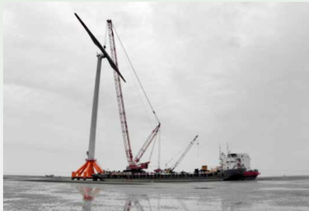
Figure 3. The largest offshore wind power installation vessel in China
