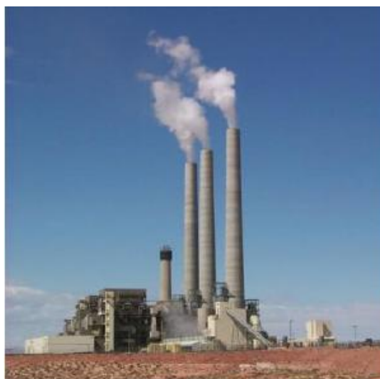
Fig. 4.2 Example photo of a thermal power plant
