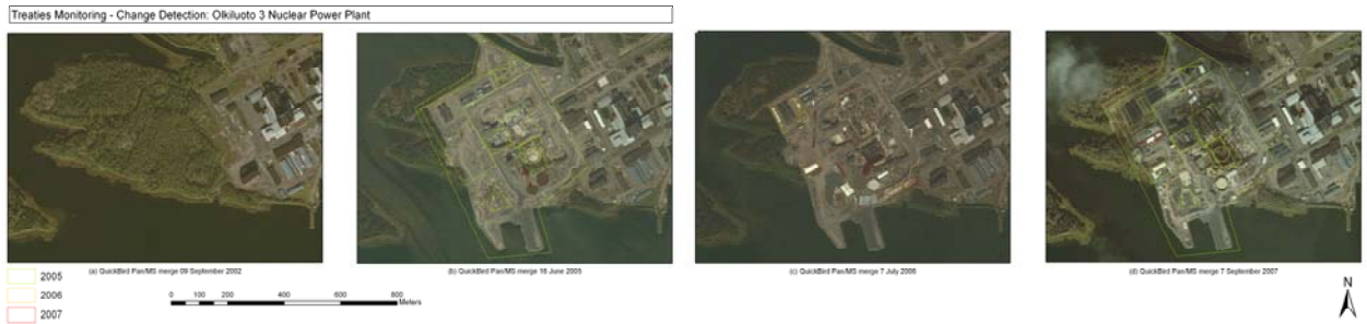
Figure 3: The four images show the site of the EPR reactor before the construction (2002) and at different instances during the construction (2005, 2006 and 2007). The images include the annotations resulting from the standard, visual interpretation carried out by an image analyst.
