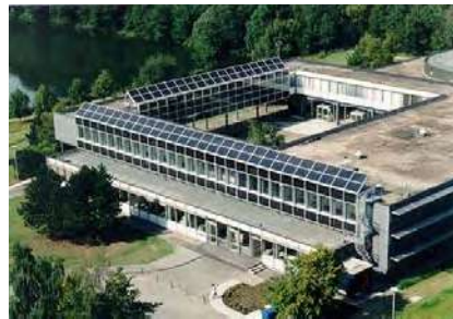
PV System on FZJ Central Library (Test of seasonal storage)
