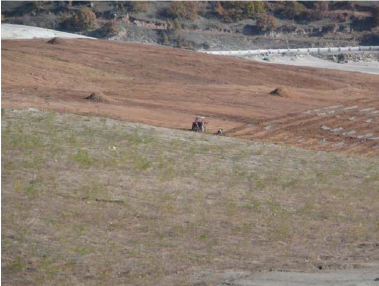
Figure 3: Flotation dump after applying of the soil and geological material
