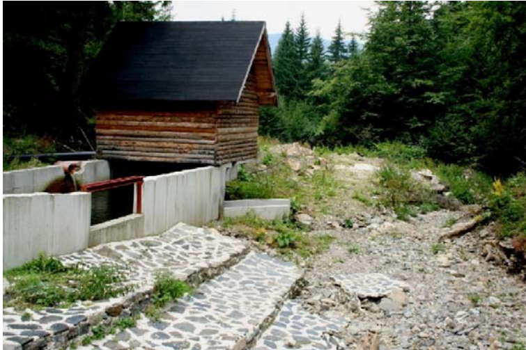
Figure 7: Lack of water in the river bed of Vrbas below the mini hydro dam and an additional water supply from unknown forest spring (red pipe)
