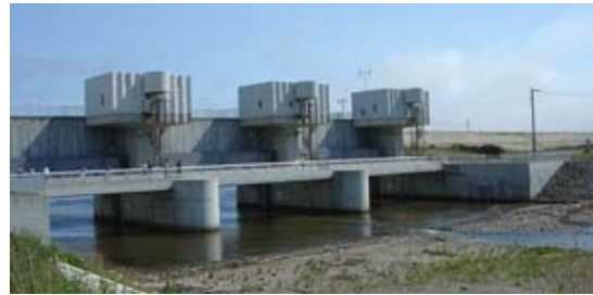
Figure 3: Water gate used on Okushiri Island.
