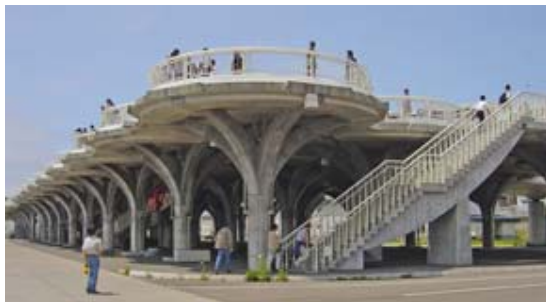
Figure 2: Elevated platform used on Okushiri Island ( http://ioc3.unesco.org/itic/printer.php?id=20 )
