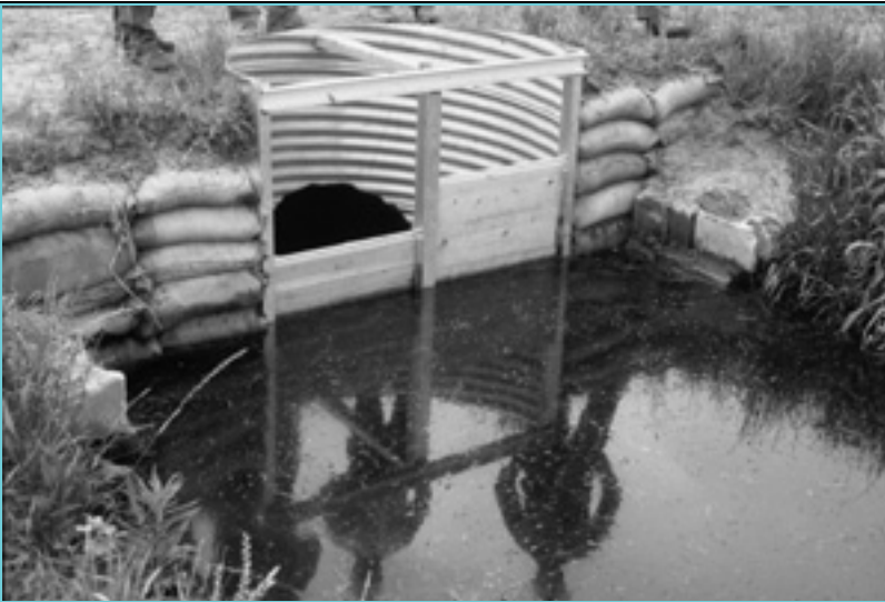
Fig. 2 Controlled drainage system showing flashboard riser ( http://www.soil.ncsu.edu/ )
