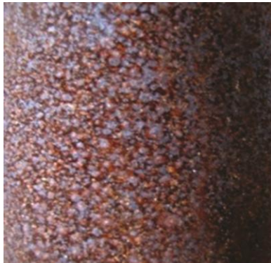
Fig. 2 — The diagram of steel tubes surface after corrosion.
