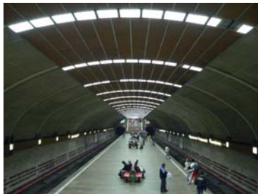
The subway in Bucharest, retrofitted by Metrorex s.a.
