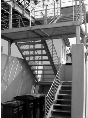
Figure 16-1: Usual metal works with steel S235JR within the limits of confidence zone 1
