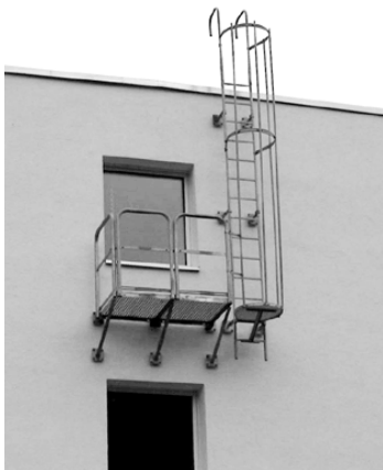
Figure 16-1: Usual metal works with steel S235JR within the limits of confidence zone 1
