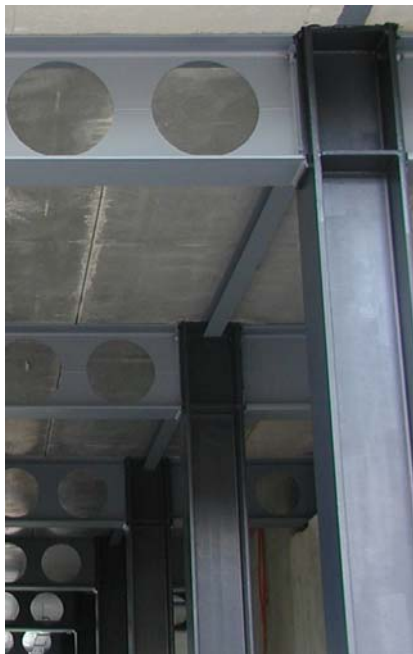
Figure 8-3: Beam to column connection
