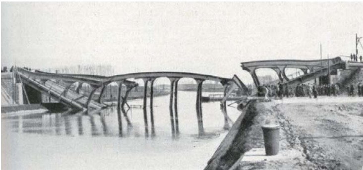
Fig. 1-1: Sudden collapse of the 1 year old roadway bridge over the Albert canal near to Hasselt due to brittle fracture, Belgium, 1938
