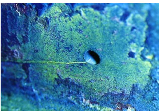
Fig. 3-13: Quality control after stop hole drilling using MPE [Lit. 13]
