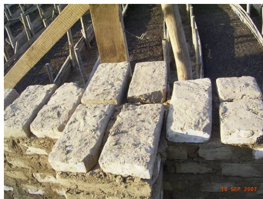
Figure 13.2 Reconstruction of an adobe wall using traditional techniques in El Carmen
