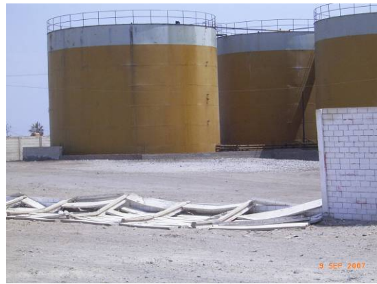
Figure 9.2 Toppled RC prefabricated perimeter walls and undamaged steel tanks along the coast near Pisco
