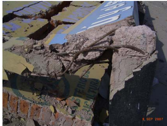
Figure 5.36 Detail of the RC columns of the Pozo Santo billboard, showing 12 mm diameter steel rebars with practically no confinement
