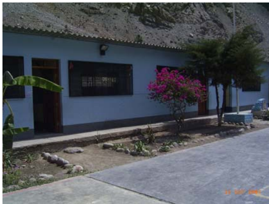
Figure 10.11 San Jerónimo (Cañete river valley): adobe school showing limited damage
