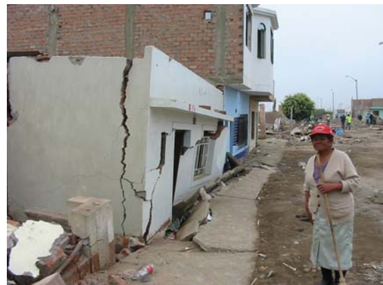
Figure 3.2 Houses in the area affected by liquefaction were mostly confined masonry
