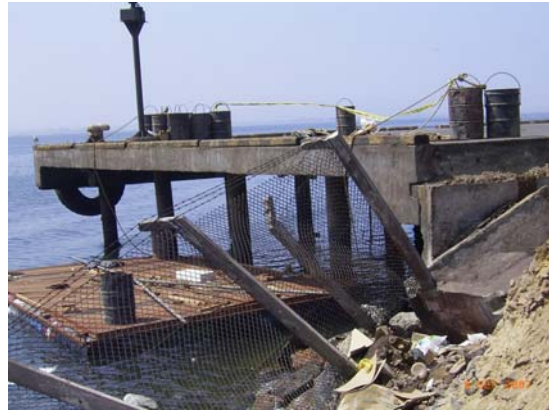
Figure 7.8 Port of San Martín: RC dock structure showing steel piles
