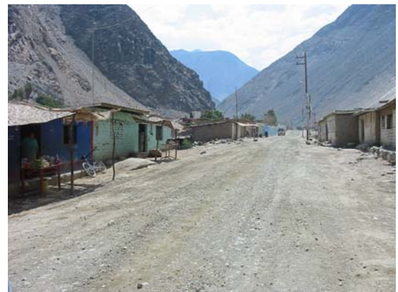
Figure 3.13 Debris fall in the mountain area along the Cañete river valley
