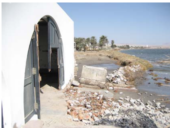
Figure 4.3 Tsunami damage at shore in front of holiday villas in Paracas
