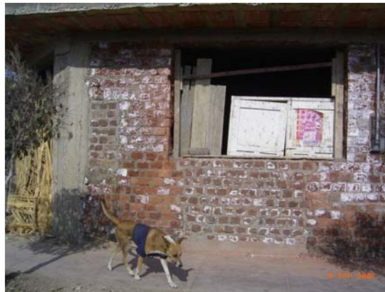
Figure 5.16 RC infilled confined brick masonry house in Guadalupe
