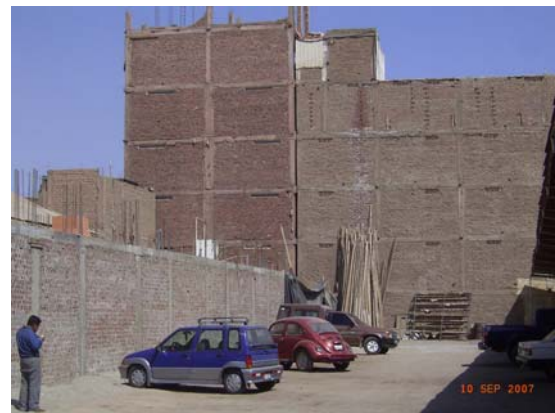
Figure 5.25 Six-storey RC confined masonry building in Ica, showing no signs of damage
