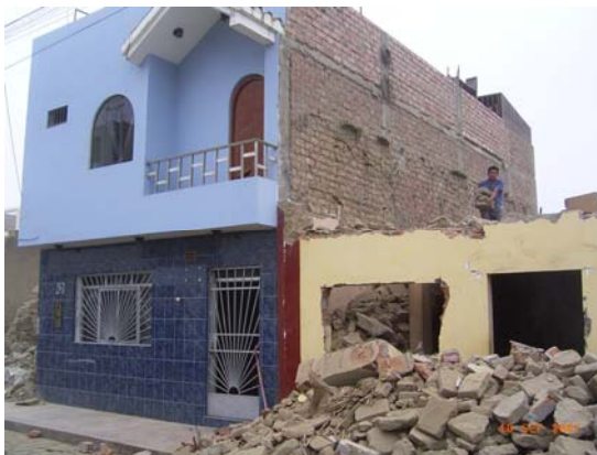
Figure 5.24 Undamaged two storey RC confined masonry building next to a collapsed adobe house in Ica
