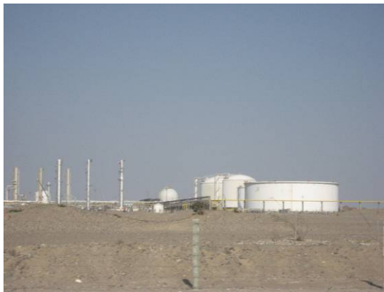
Figure 9.1 Industrial facilities along the coast near Pisco
