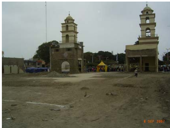
Figure 5.38 Location of the collapsed church in Pisco after demolition and debris removal
