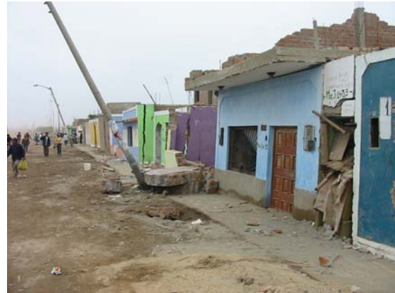
Figure 3.4 Street lamps toppled at the base up to approximately 50° with the horizontal plan
