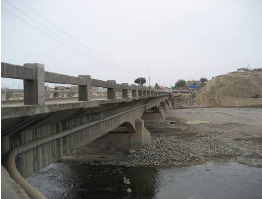
Figure 6.4 Huamaní Bridge along the Pan-American Highway
