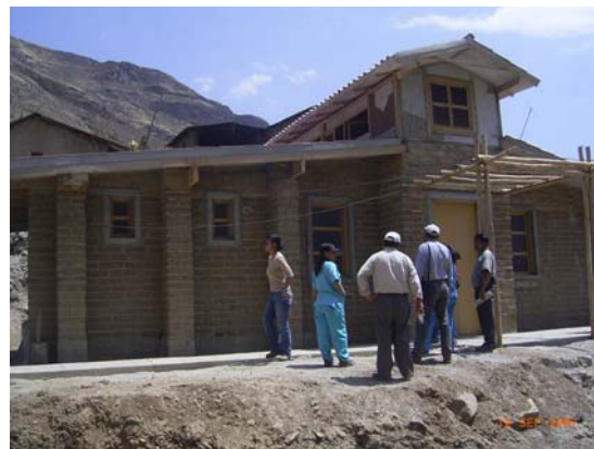
Figure 5.22 Adobe house in Huangáscar built by JICA and designed for earthquake resistance
