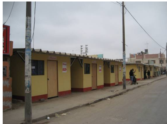
Figure 12.4 Temporary accommodations in Pisco (made of steel/ aluminium sheets)
