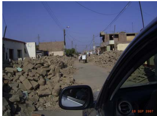
Figure 5.4 Debris of collapsed adobe houses in Ica
