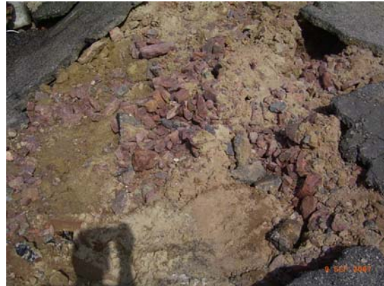
Figure 7.4 Port of San Martín: fill material of the paved access to the dock structure
