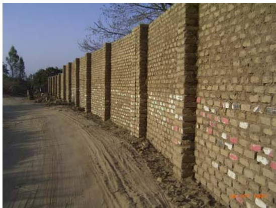
Figure 5.10 Freestanding adobe wall near Guadalupe with lateral supports (or machones )
