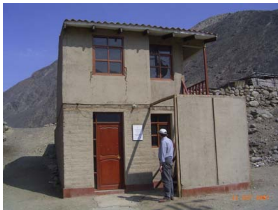
Figure 5.21 Two-storey adobe (and quincha at second storey) built by JICA in Zúñiga for earthquake resistance
