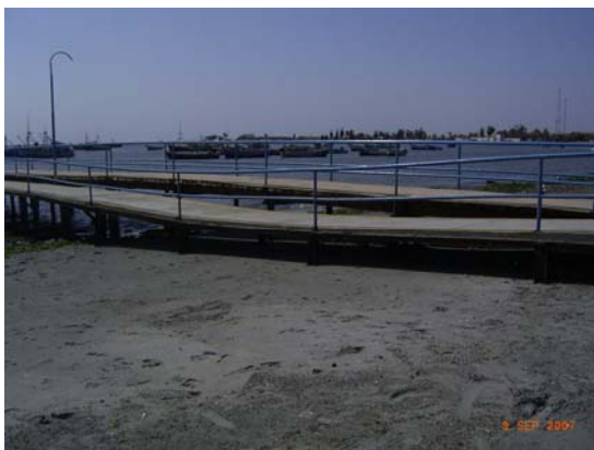
Figure 7.11 Dock structure in Paracas
