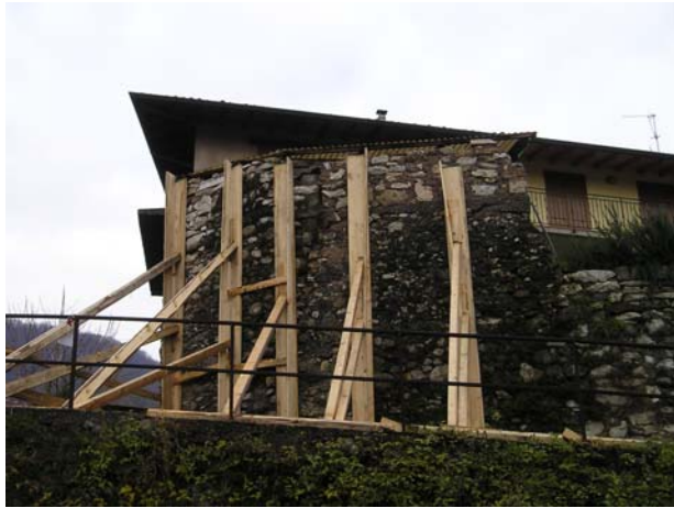
Figure 5.5. Safety intervention on a stone masonry wall
