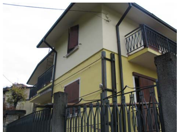
Figure 5.10. Safety intervention in Collio
