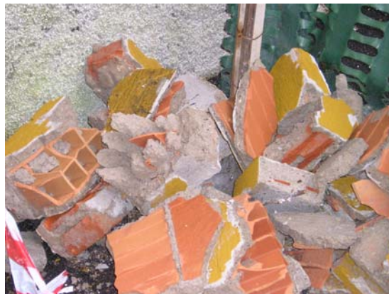
Figure 4.21. Hollow bricks used in Pompegnino
