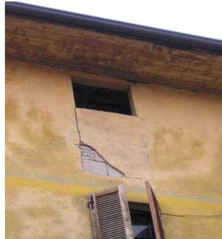
Figure 4.2. Separation of infills in Collio
