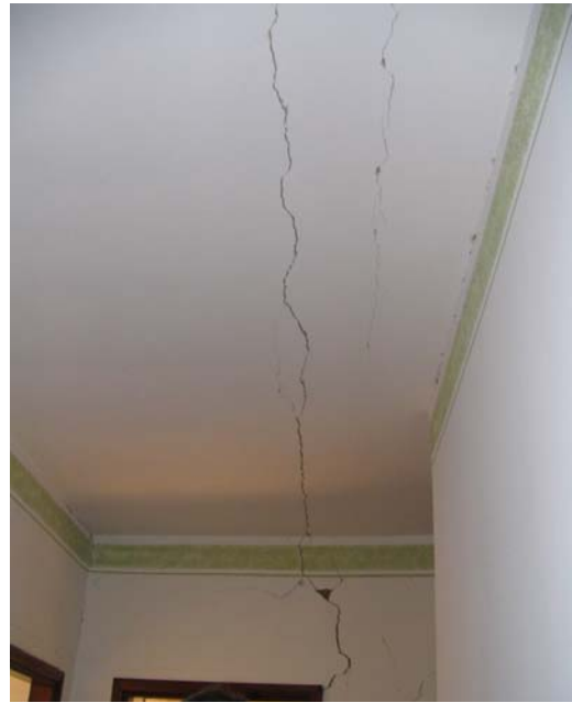
Figure 4.10. Renovated house in Pavone
