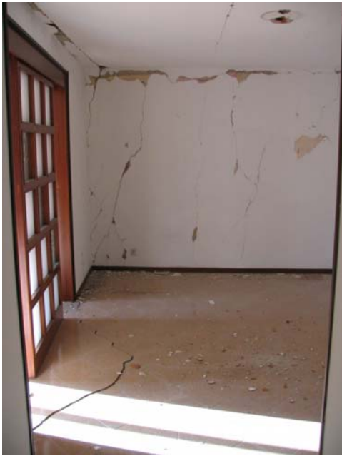
Figure 4.9. Renovated house in Pavone
