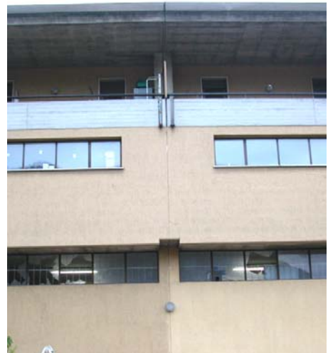
Figure 3.7. Separation joint in RC building
