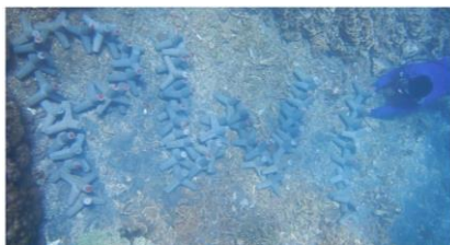
Gambar 8. Proses Penenggelaman Puzzle Tetrapod (Dok, 2019)
