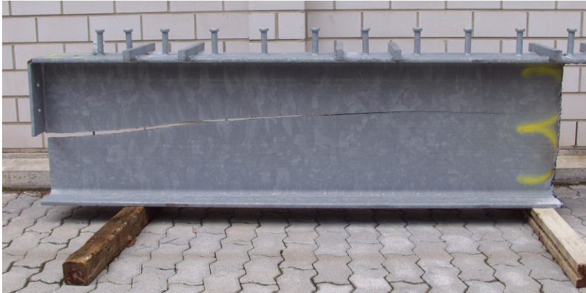
Fig. 7-1: Example of cracks from zinc coating by hot dip galvanizing
