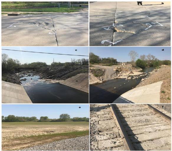
Figure 7. Field photos showing mass wasting in limestone terrain. (a and b) the pavements show the crack on the pavement as a result of differential settlement of the compacted soils; (c and d) show sides of the river channel falling into the river; (e) Sink hole shows subsidence in the topsoil which is indicative of an incompetent subsurface layer. (f) mud cracks evident along the Buzzi Cem rail tracks evidencing flooding of tracks.
