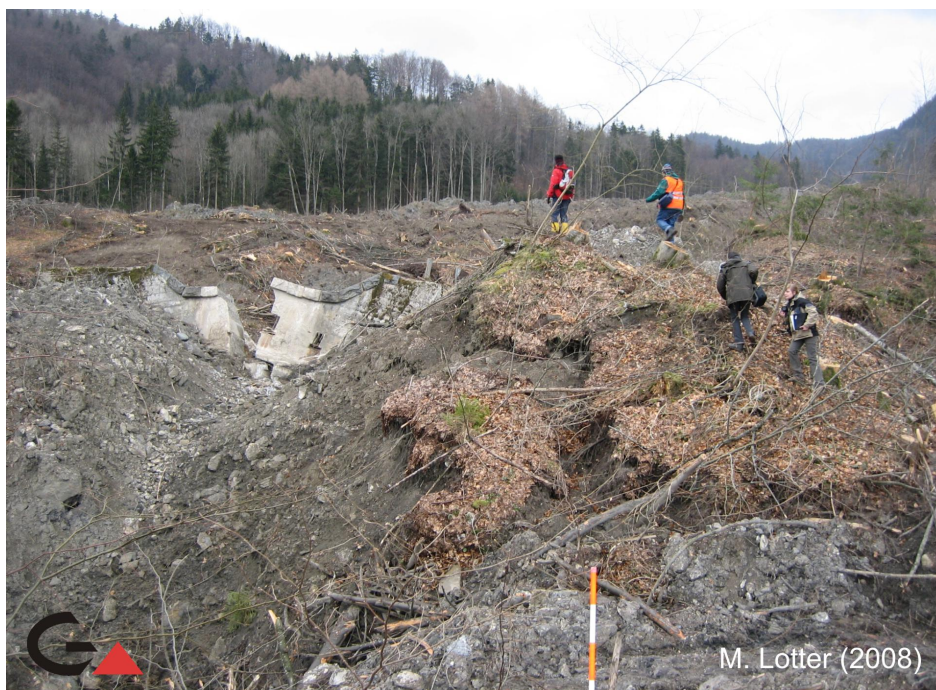
Fig. 6. Landslide of Gschlifgraben. Completely destroyed dams are shown in the foreground. (Source: M. Lotter, 2008 – Archive of GBA)
