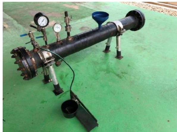
Gambar 3. Instalasi Manifold Hydrotest Temporary Clamp 8 inch
