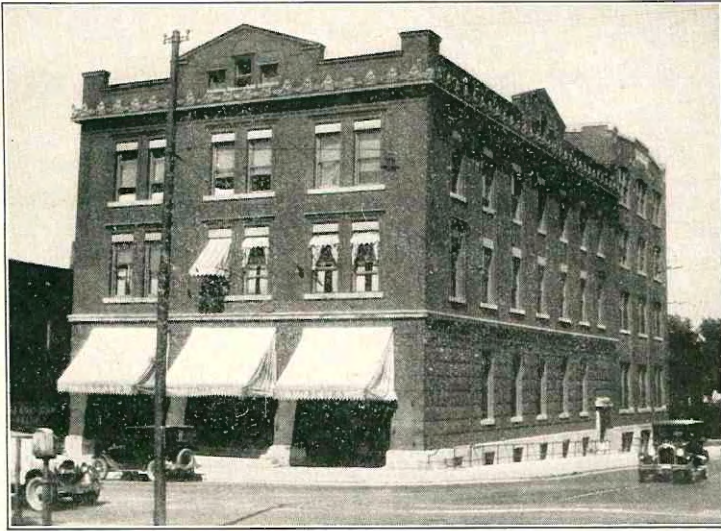
AUGUSTANA BOOK CONCERN Building Unit Completed in 1912
