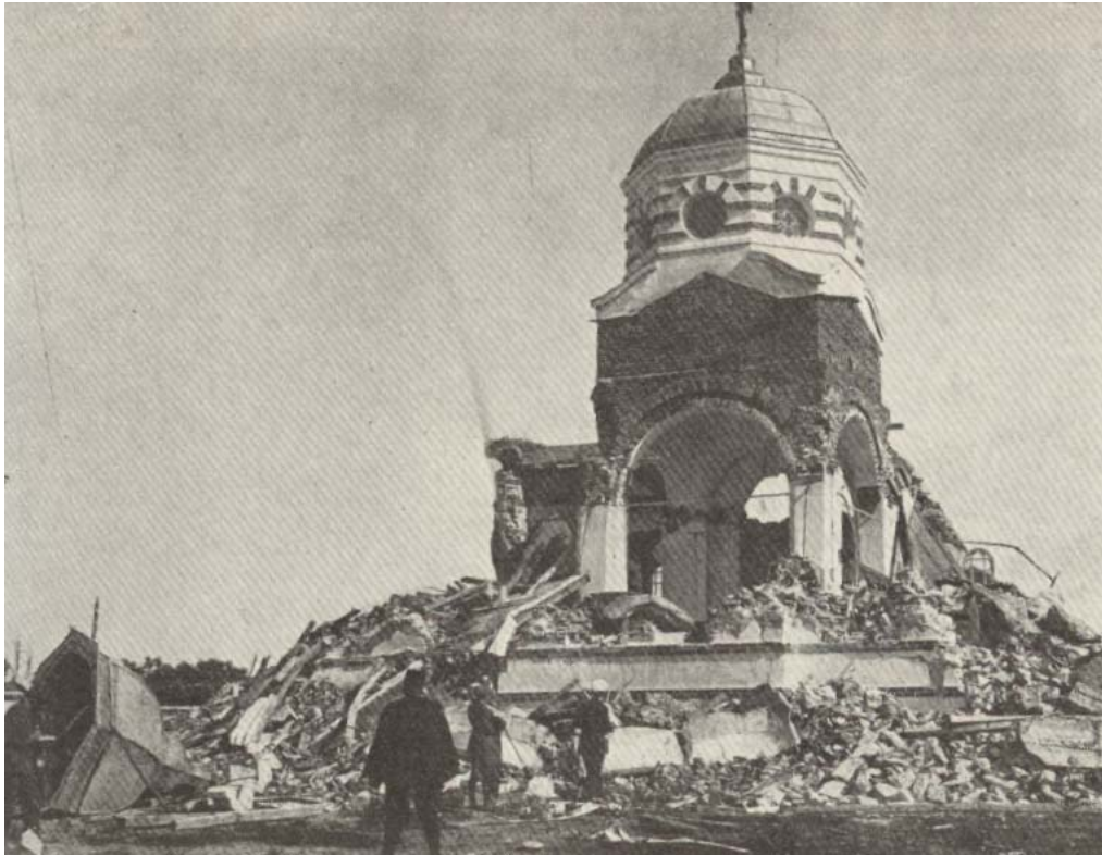
Figure 2: Destroyed church after the 1928 earthquakes in Bulgaria (M7.0 and 6.8)
