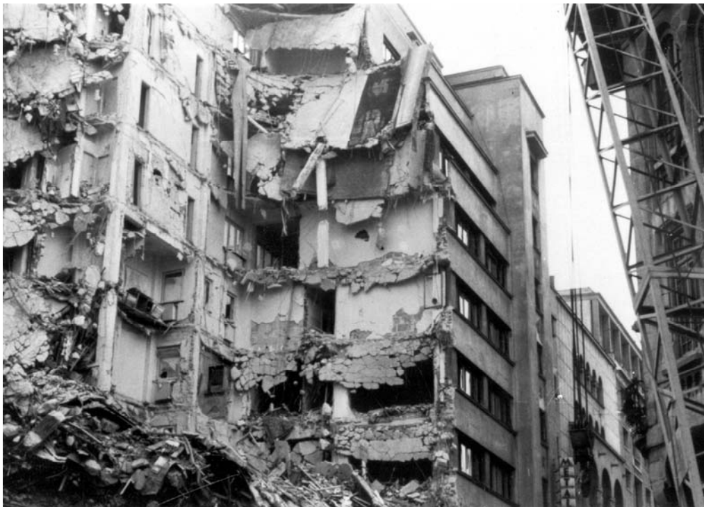
Figure 3: Partially collapsed reinforced concrete frame and masonry wall office and apartment buildings in Bucharest, Romania after March 4, 1977 earthquake. Photo by C. Rojahn 1977, U.S. Geological Survey Photographic Library,
