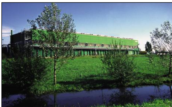
Figure 7: ECODECO SRF Processing plant, Milan, Italy
