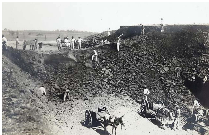
Figure 1 – Cutting excavation, stretch Dois Córregos-Jaú, 1935 (new line), 1935 Source: São Paulo State Public Archive.
