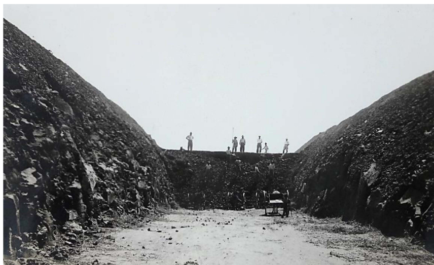
Figure 2 – Cutting excavation, stretch Dois Córregos-Jaú, 1935 (new line), 1935 Source: São Paulo State Public Archive.
