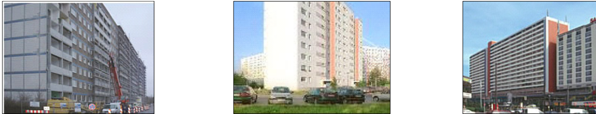
Figure 3.3 Panel buildings especially erected in the eastern European states Source: [WETZEL & VOGDT 2005]
