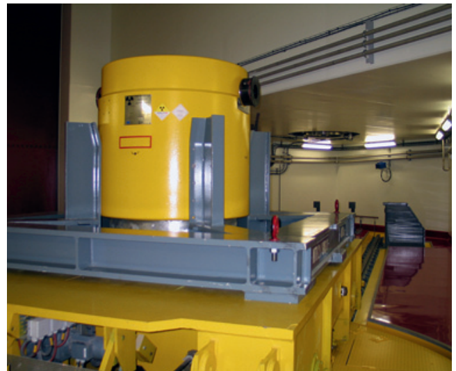
Figure 10 - MTR2 container at COVRA on its way to the docking station underneath the hot cell of HABOG
