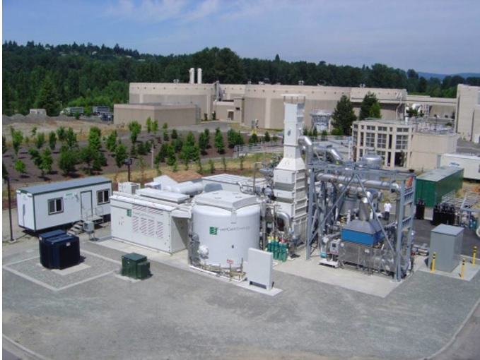
Figure 2. King County Power Plant (Courtesy of FCE)
