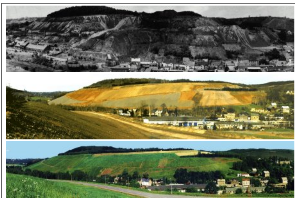
Figure 15: The progress of remediation over a 20 year period at one of the Wismut uranium mining sites gives an indication of the amount of energy expenditure required.
