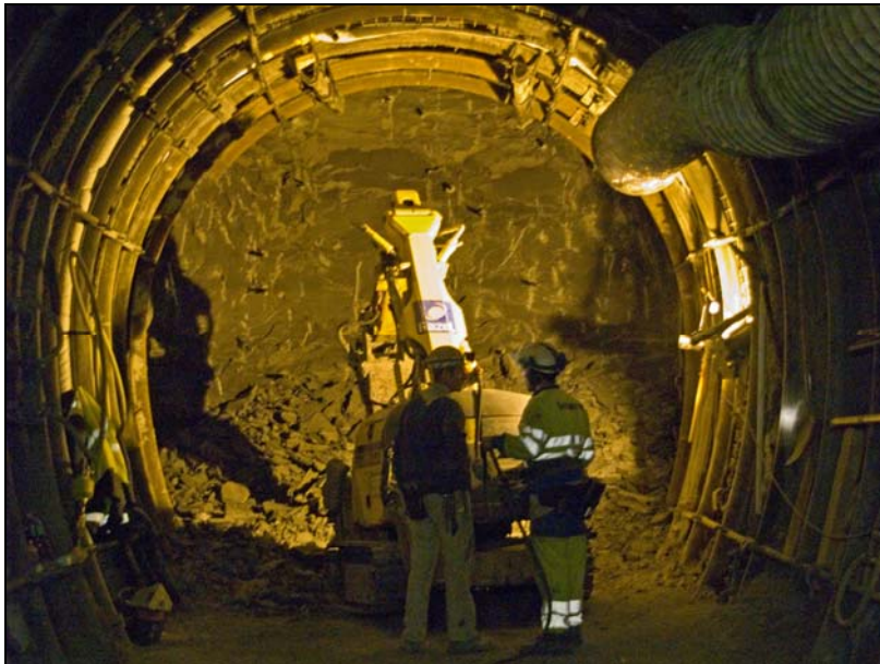
Figure 11: Typical mine face, showing excavating machinery and steel liners.
