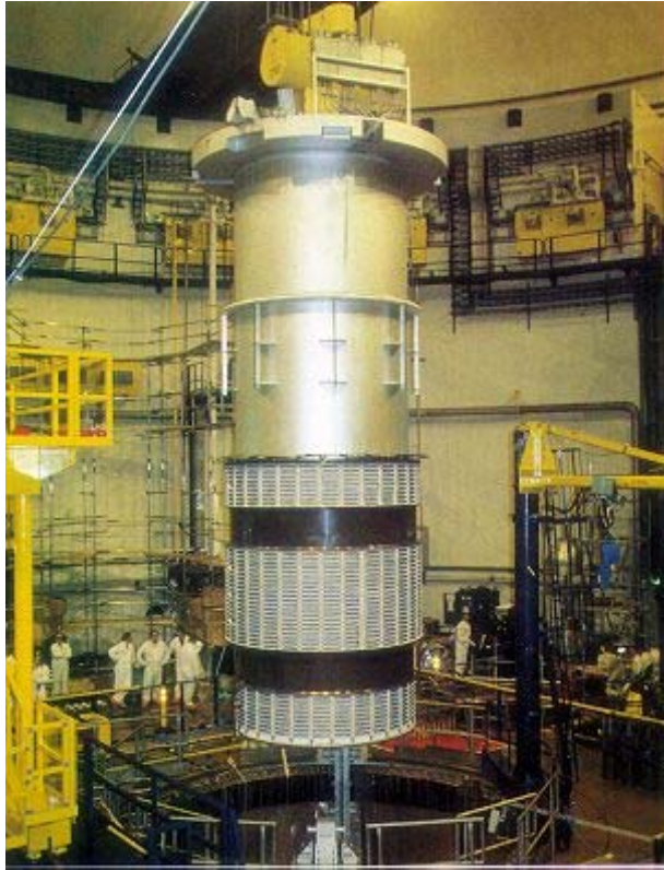
Fig. 5.5 Photo of the SKODA annealing device before loading into the RPV
