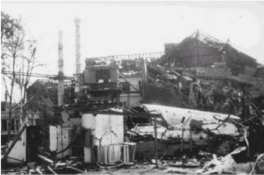
Figure 10 – Factory after rupture and explosion of a hydrogen storage tank [12]
