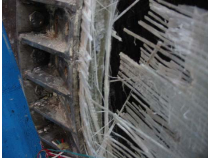
Figure 144 Final extraction of tower base from steel anchorage ring.
