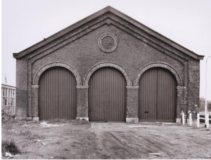
Figure 12: Plate 2, Harlingen, NL 1963. Photograph by Bernd and Hilla Becher from the book Industrial Façades 1982. Courtesy of MIT Press, Schirmer/Mosel Verlag.
