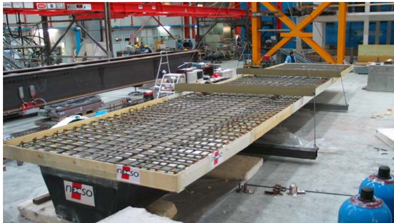
Figure 30 Reinforcement of RC deck.
