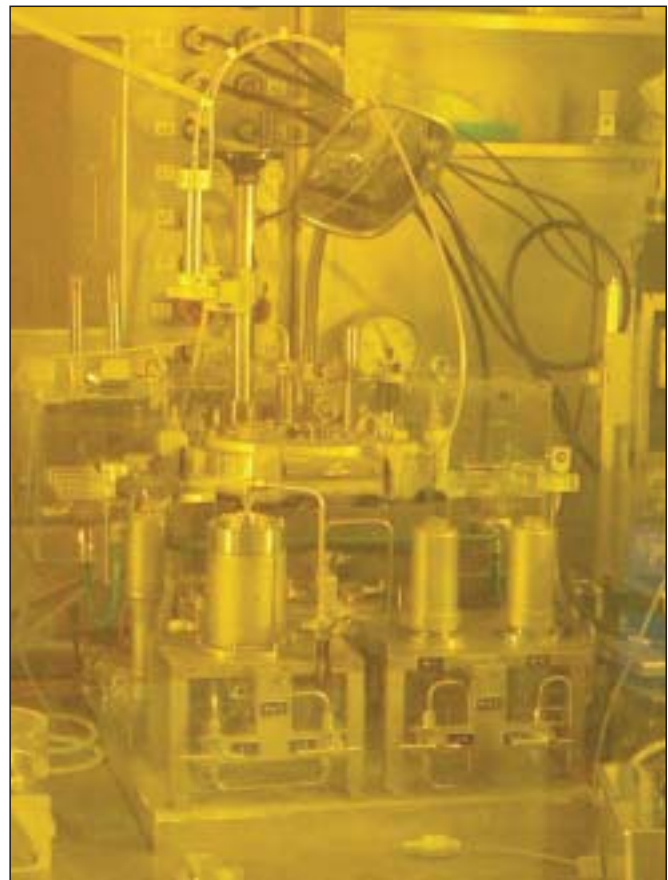
Fig. 3.6 View of the new high temperature oven facility after installation in the hot cell 106.
