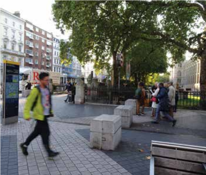
Security retrofit: Granite bollards have appeared in key locations, such as the intersection with Cromwell Gardens to provide a physical barrier, protecting crowded pedestrian areas around the museums from the threat of terrorism.
